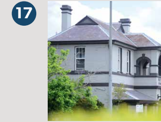
Fry Bros Building & Stone Cottage
